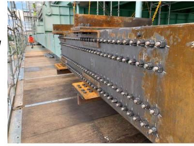
Offset Plate to clear Fracture and Ex Splice.
